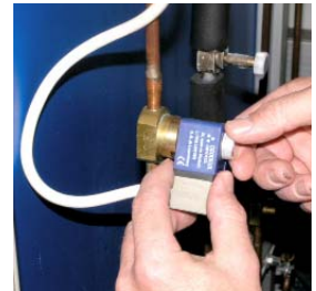
4. Mounting of the coil
