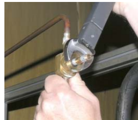
3. Mounting of valve cartridge
